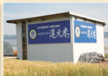
A large sign put up on the work shed to appeal to neighboring farmers. 作業小屋に取り付けた看板で近隣の農家にアピール
